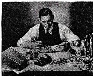
This portable electroplating outfit makes it possible to electroplate objects without subjecting them to the usual plating tank. Objects fastened down can be replated without being removed. The unit uses a brush as an anode, which spreads the plastic plating solution.
