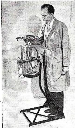
This new clamp device for lawn mower repairing allows the worker to have free use of both hands, by holding the mower rigid in any position desired. The clamp suspends the mower at three points between the roller and tie-rod, with a snap-hook around the center of the tie-rod. The various positions of the mower can be changed at will without removing it from the clamp.
