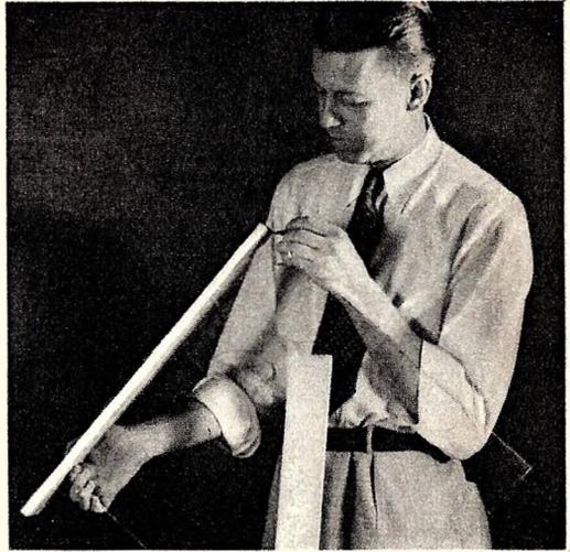
**TRAY FOR DEVELOPING LARGE PRINTS.** Prints of large size can be developed in a tray made of an old window pane with rabbeted pieces of wood attached to each side. The glass bottom and wood sides should be given two coats of asphalt varnish before use.
