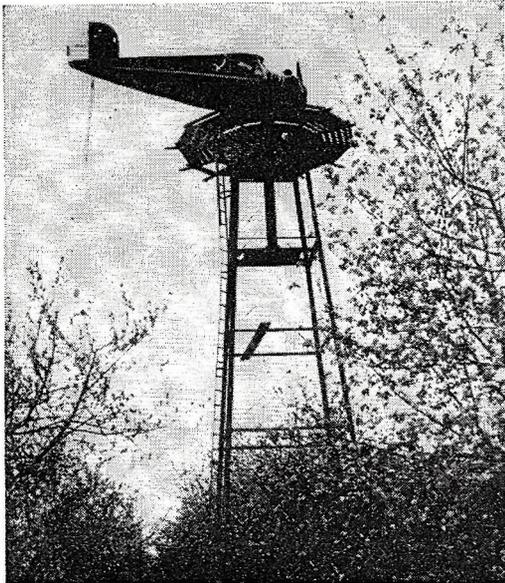
Mounted atop a 40-foot steel tower on a fruit farm near Painesville, Ohio, an obsolete wingless airplane is being used to prevent dew from forming on trees and freezing, thus damaging the orchards. When the temperature falls a bon-fire is lighted, sending up heated air which is blown over the orchards by the propeller of the airplane.
