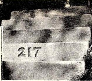
Numbers can be indented into a concrete block which can be set into a step, makes a lasting arrangement. Before pouring concrete, coat the wooden numerals with a layer of oil.
