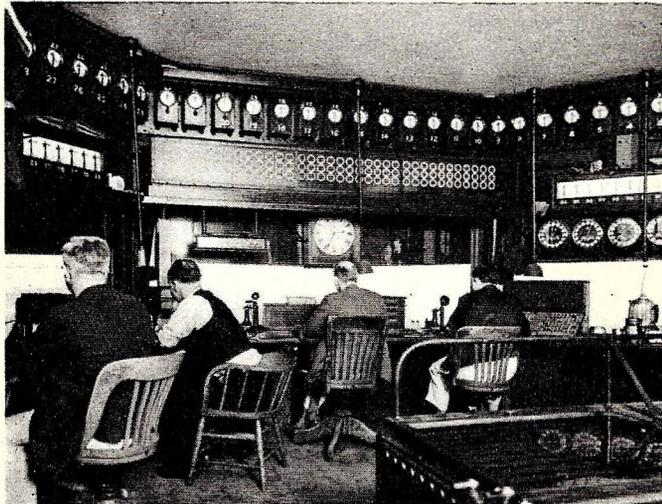
Left—This shows the director's desk in the interlocking tower of the Washington, D. C. terminal. Dials above repeat signals in the yard outside. Above: Showing track control panel of the terminal.
